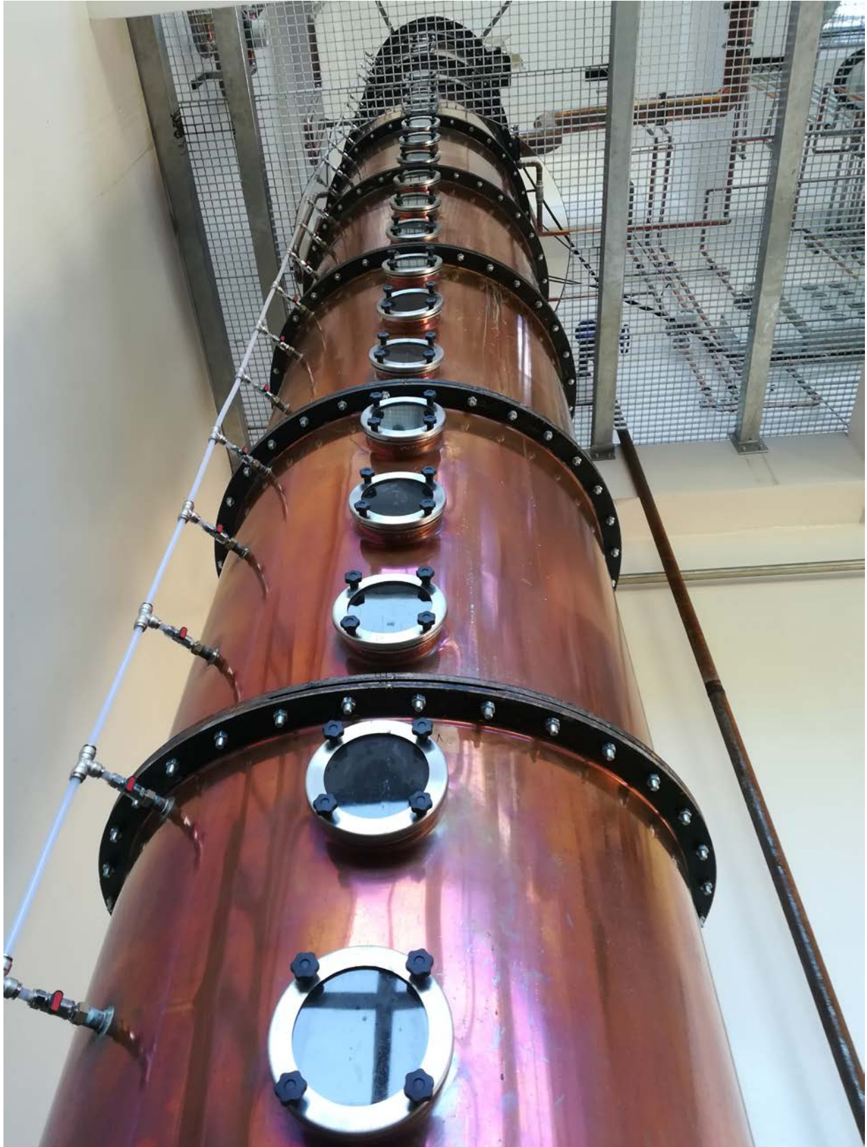
New distillation column, 2018.
